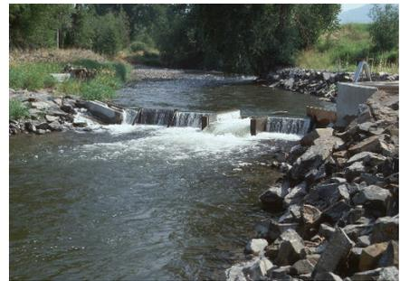
Reduced flows, increased temperature, nutrients & algae can lead to low DO measurements. Investigate opportunities for aerating water by having it tumble over rocks, weirs, etc. Minimize ‘dirty’ tailwater returning to the system.
